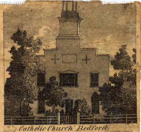
Catholic Church Bedford.
