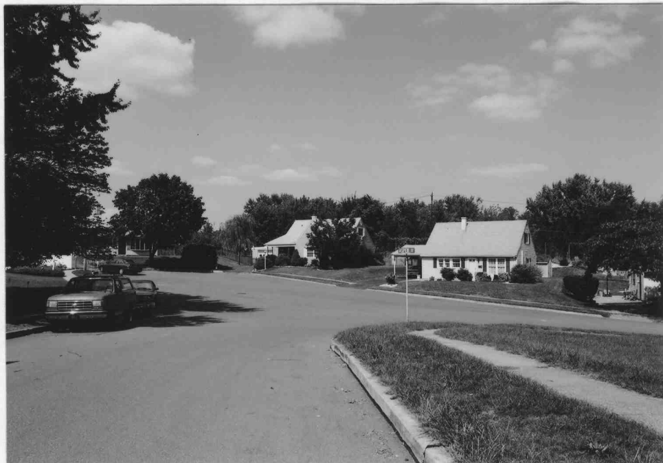
Oak Hills Subdivision: Photograph 7—Looking northwest at the corner of Aspen Street and Pine Street within the Oak Hills 2 section.
