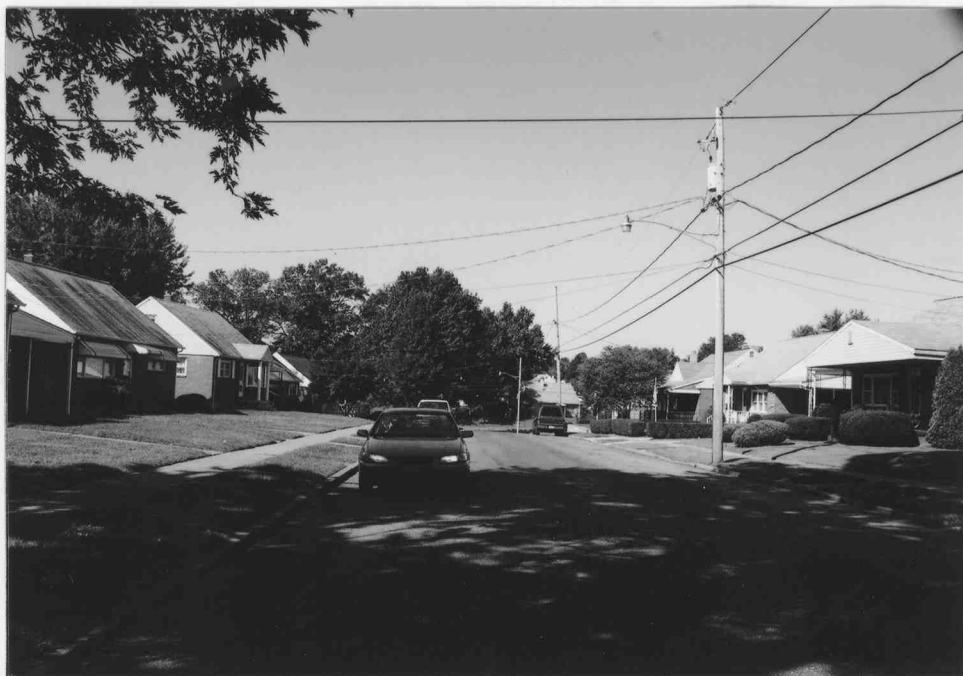
Oak Hills Subdivision: Photograph 16—Looking southwest along Ridge Avenue in the Oak Hills 1 section.
