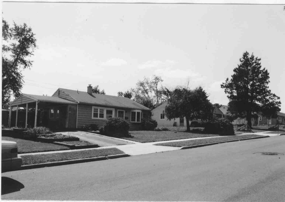
Oak Hills Subdivision: Photograph 13—Looking southwest along Catalpa Street in the Oak Hills 2 section.
