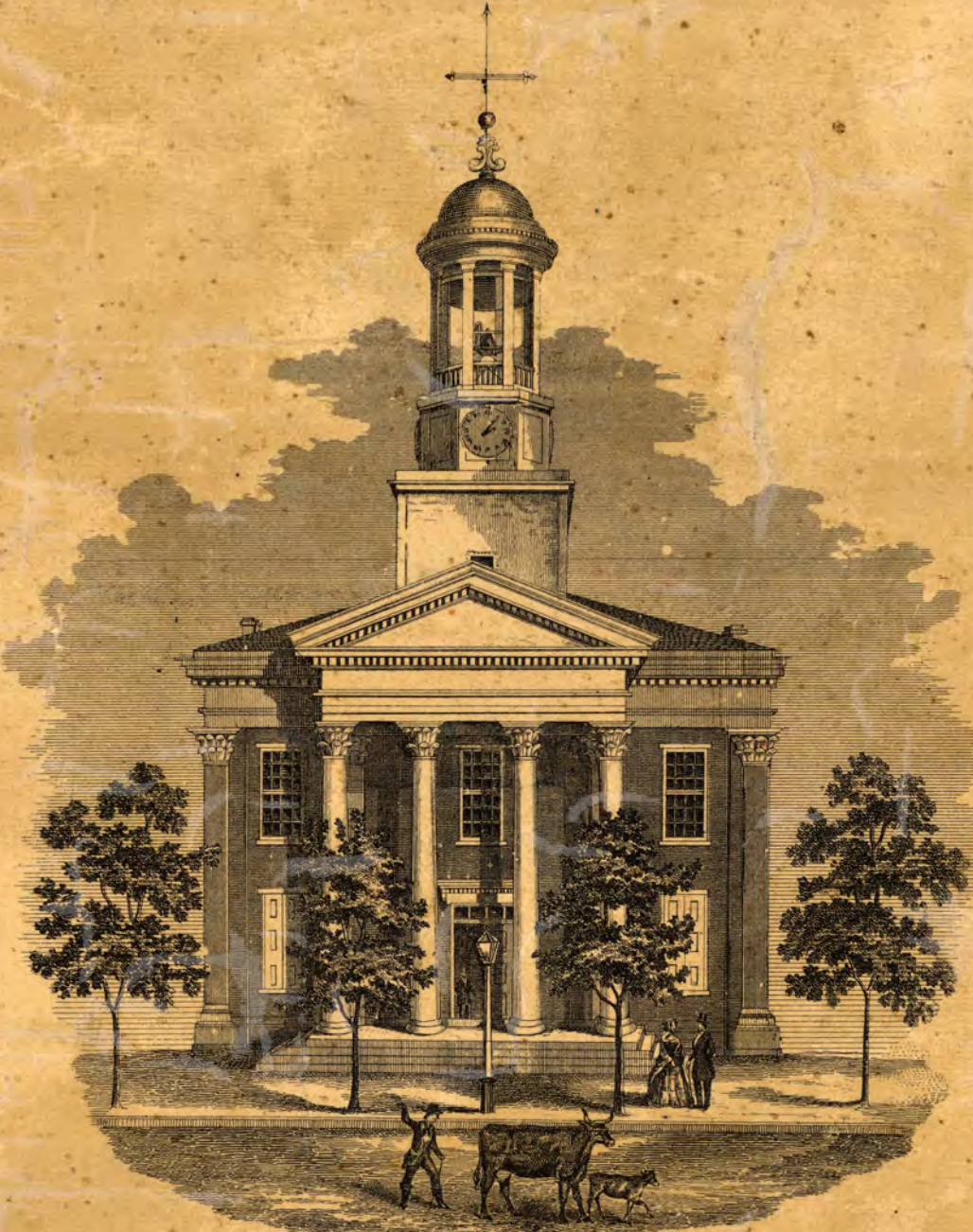
COURT HOUSE Carlisle.
