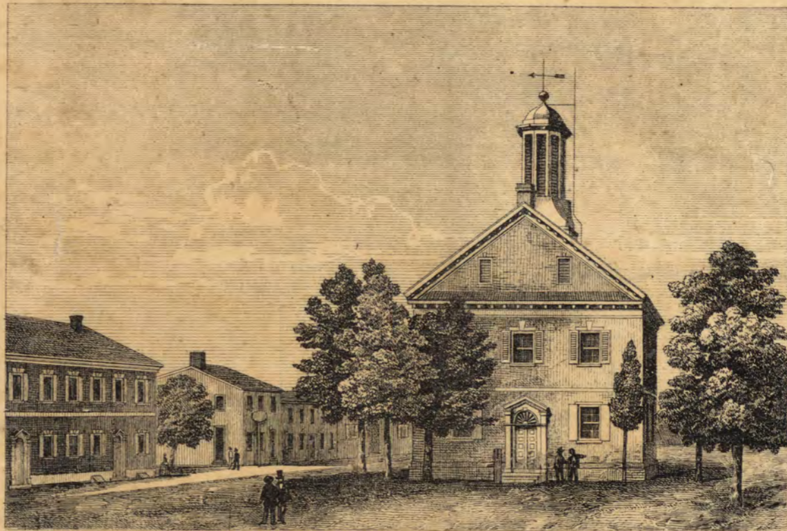
NORTHUMBERLAND COUNTY COURT HOUSE. Sunbury, Pa.
