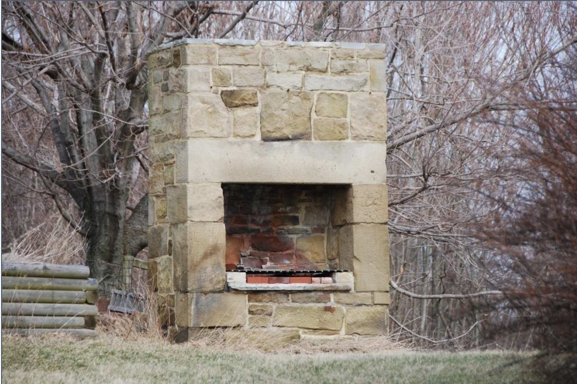
#803100—Mary Hoge Rd., Waynesburg, Whiteley Township Greene County. An outdoor bake oven from the 19 th century.
