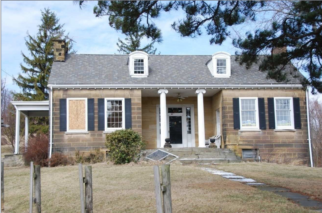
#803100--333 Mary Hogue Rd, Whiteley Township, Greene County (front façade). Recessed front porch (portico in antis) adorned with Ionic columns framing front entrance, broken transom lights, paired segmental dormers, end chimneys, slight eave over hang boxed with dentils.
