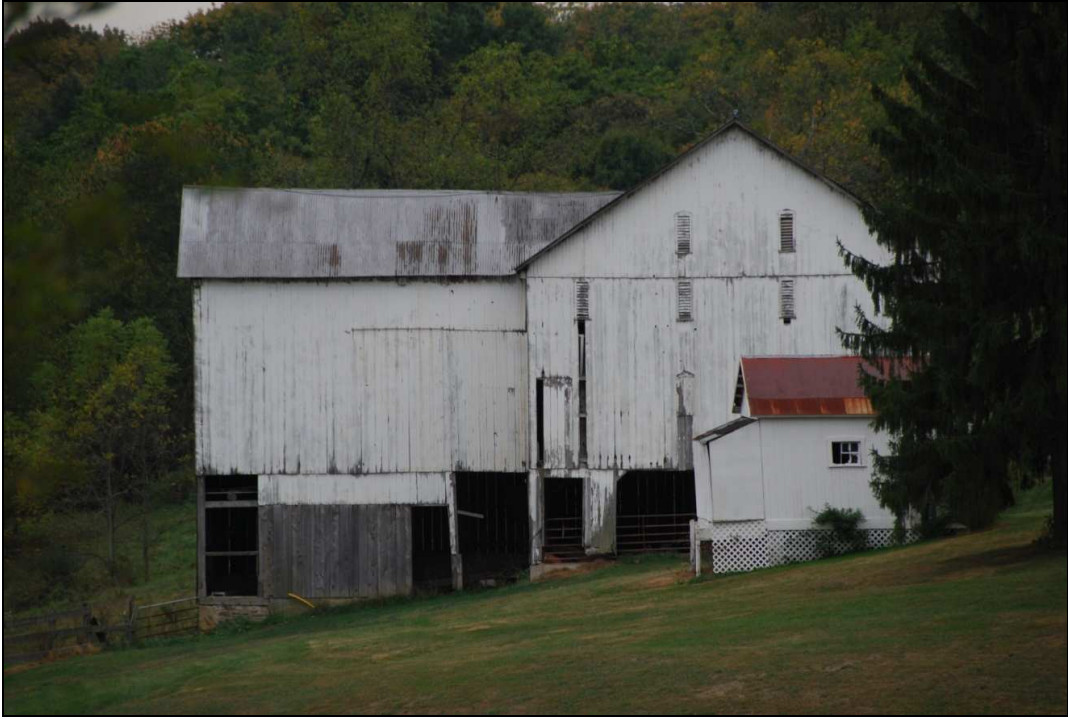
#802487—4051 Jefferson Ave., Avella, Hopewell Township Washington County. Example of a Three Gable Barn, this one is tee-shaped.
