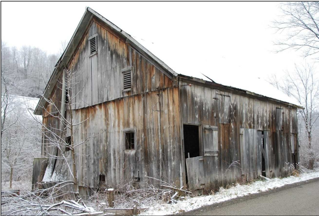
#802874—Hargus Rd., Holbrook, Jackson Township, Greene County. An example of a sheep barn with hay slide, unfortunately the slide was unable to be photographed.
