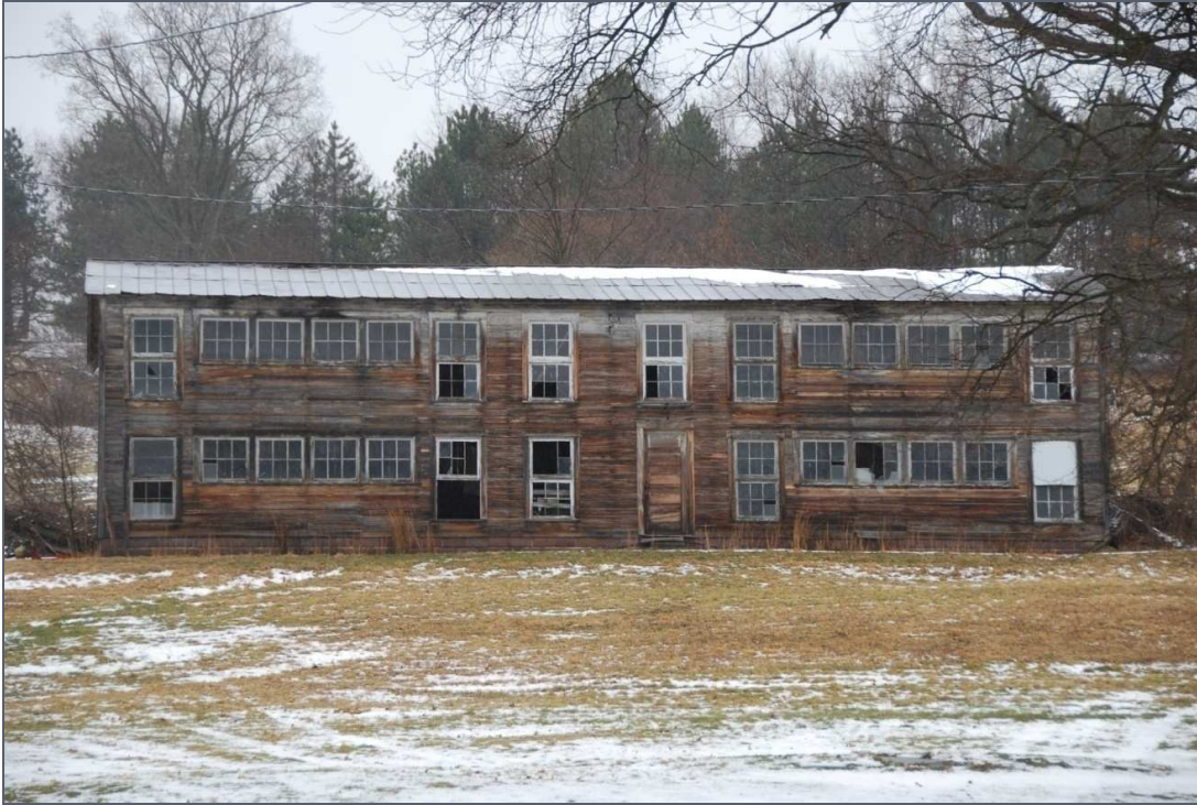
#803083—446 Garards Fort Rd., Waynesburg, Greene Township Greene County - An early 20 th century multistory poultry house
