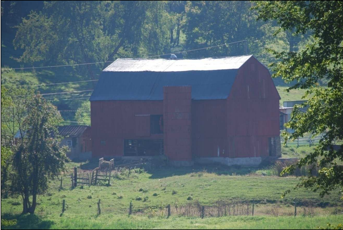
#802319—30 Weizen Rd., Coal Center, West Pike Run Township, Washington County. An example of a large Foundation barn with a gambrel roof. Notice how all the ground on the rear of the barn is completely flat with no evidence of any elevation.
