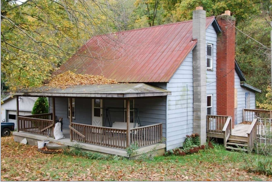
#802501—512 Poplar St., Avella, Buffalo Township, Washington Township.
