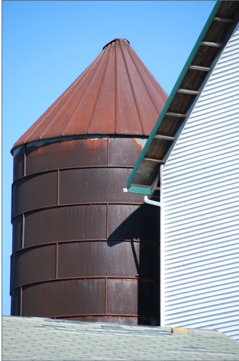
#802050—478 Midway Candor Rd., Burgettstown, Robinson Township Washington County. A steel silo.
