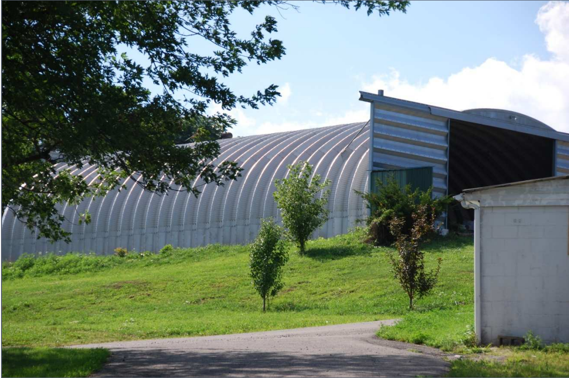
# 802112—4297 Finley Elemara Rd., Finleyville, Union Township Washington County. A Quonset machine shed.
