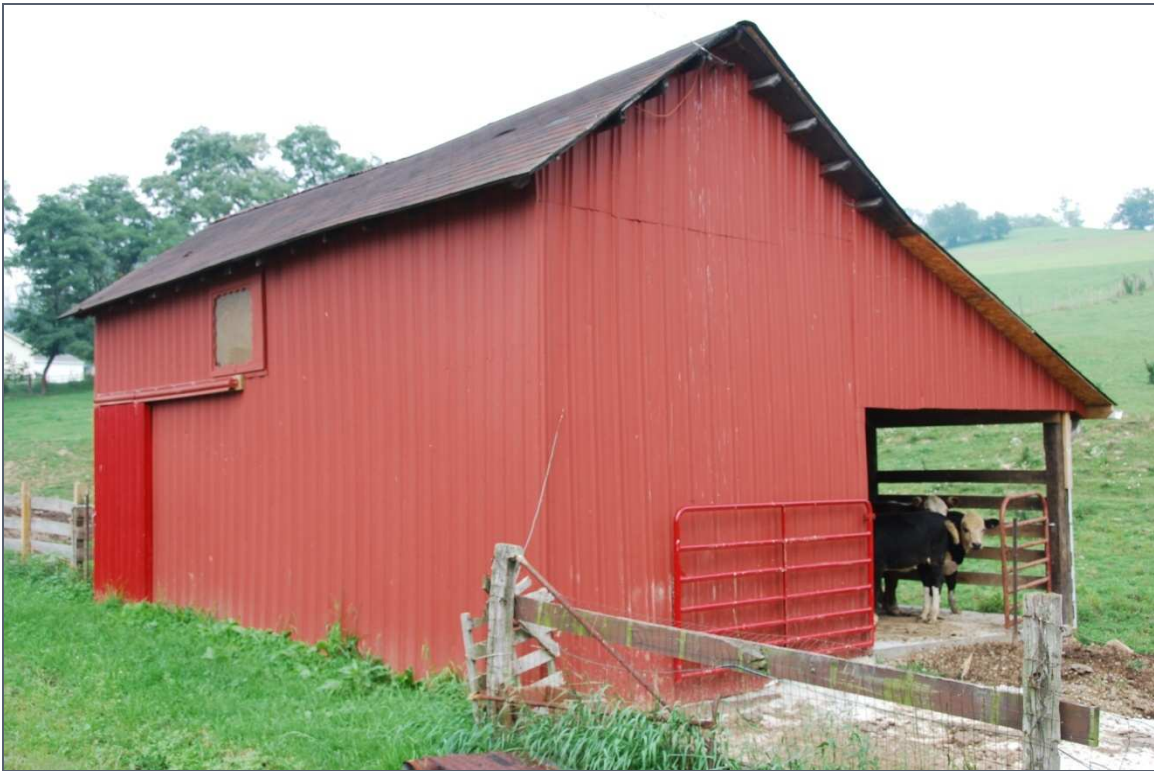
#802010—123 Beechnut Rd., Hickory, Mount Pleasant Township Washington County. A gable roof loafing shed.
