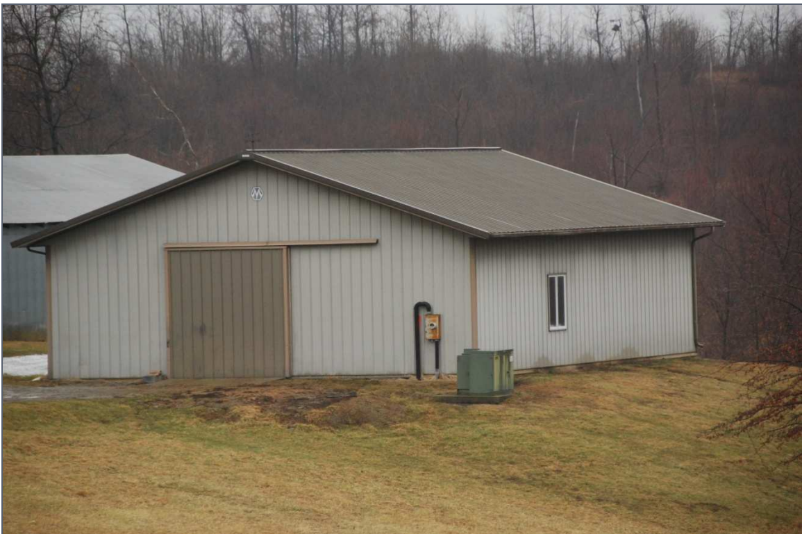
#803059—136 Colvin Rd., Greensboro, Monongahela Township Greene County. A late 20th century machine shed.
