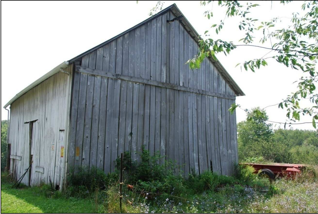
#802029—Purdy Rd., Burgettstown, Hanover Township Washington County. A simple English Barn.
