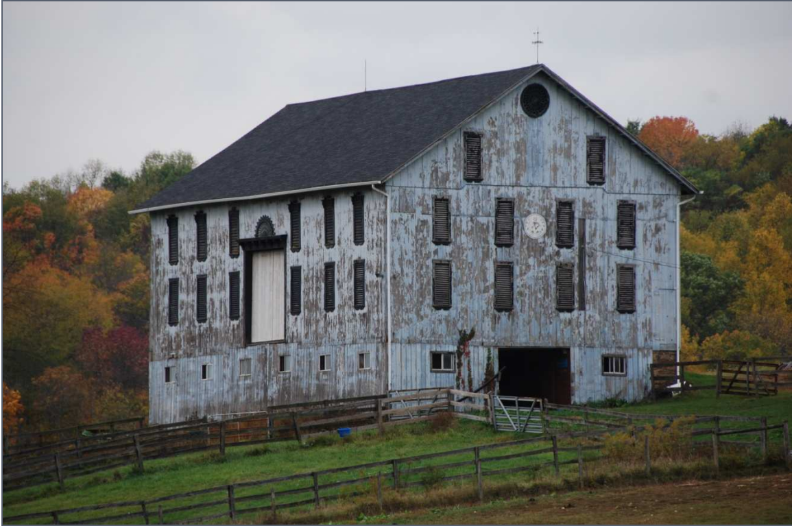
#802565—619 Pleasant Valley Rd., Washington, Buffalo Township Washington County. Basement barn with gable peak woodwork design and lowered window vents.
