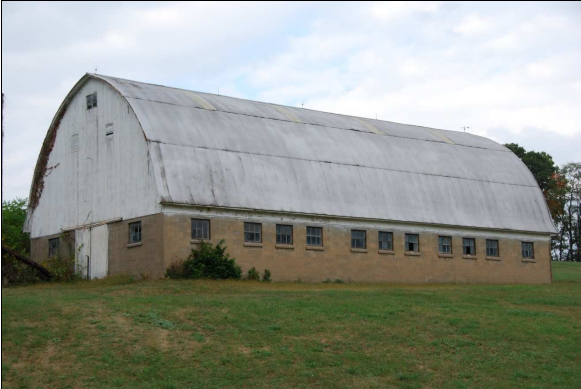
#802488—2217 Brush Run Rd., Avella, Hopewell Township Washington County. Example of a 1930's era Wisconsin Dairy Barn
