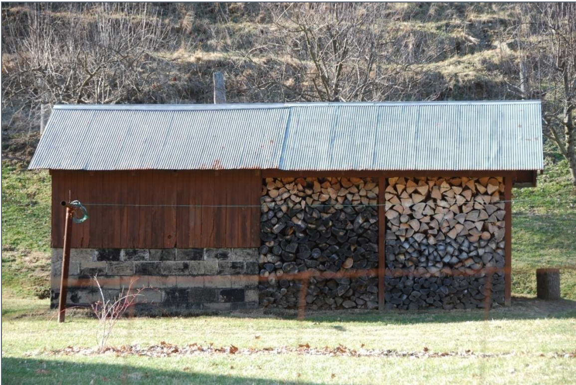
#802825—391 Morford Rd., Aleppo, Springhill Township Greene County. A wood shed attached to another structure.
