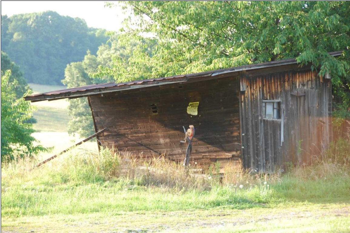
#802069—26 Covered Bridge Rd., Burgettstown, Smith Township Washington County. A late 19 th century slaughter house.
