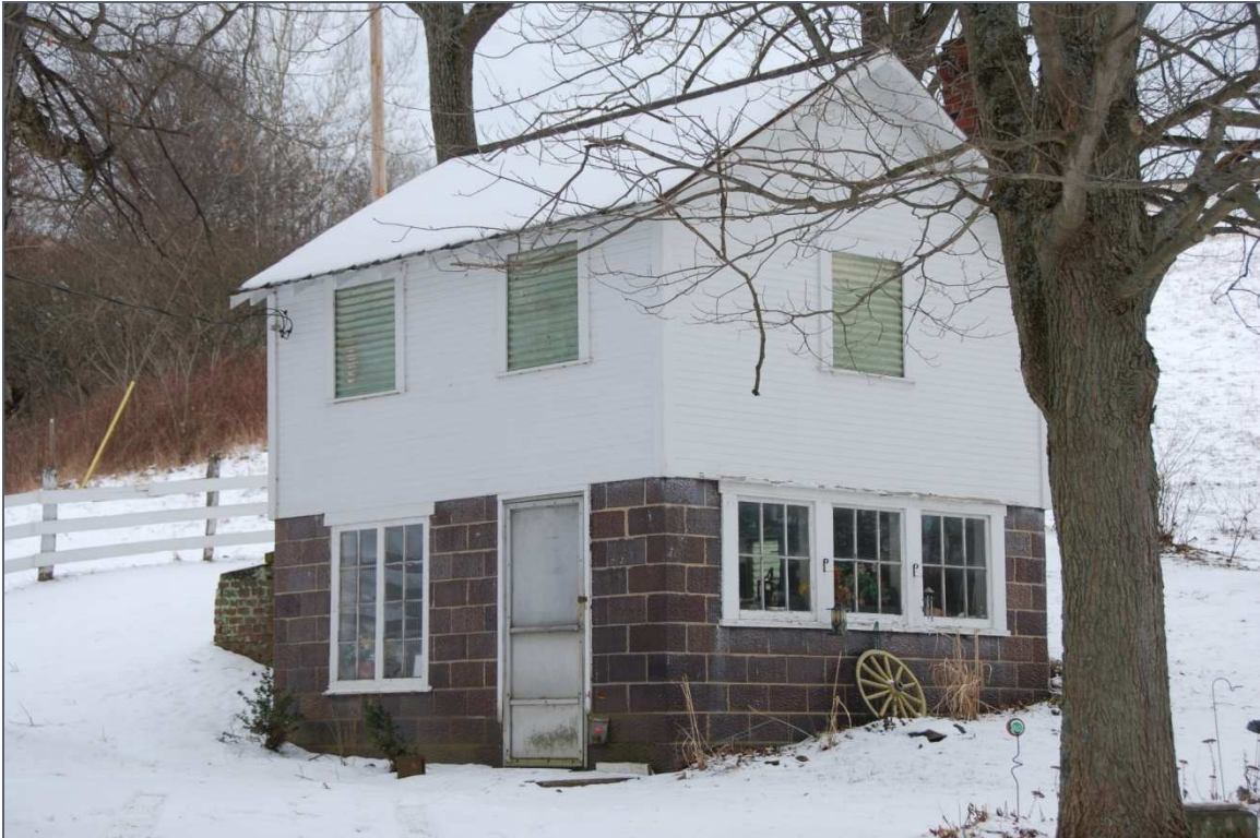
#802682—238 Walnut Valley Rd., West Alexander, West Finley Township Washington County. A dairy kitchen dating from the early 20 th century that includes an ice house on the ground floor.
