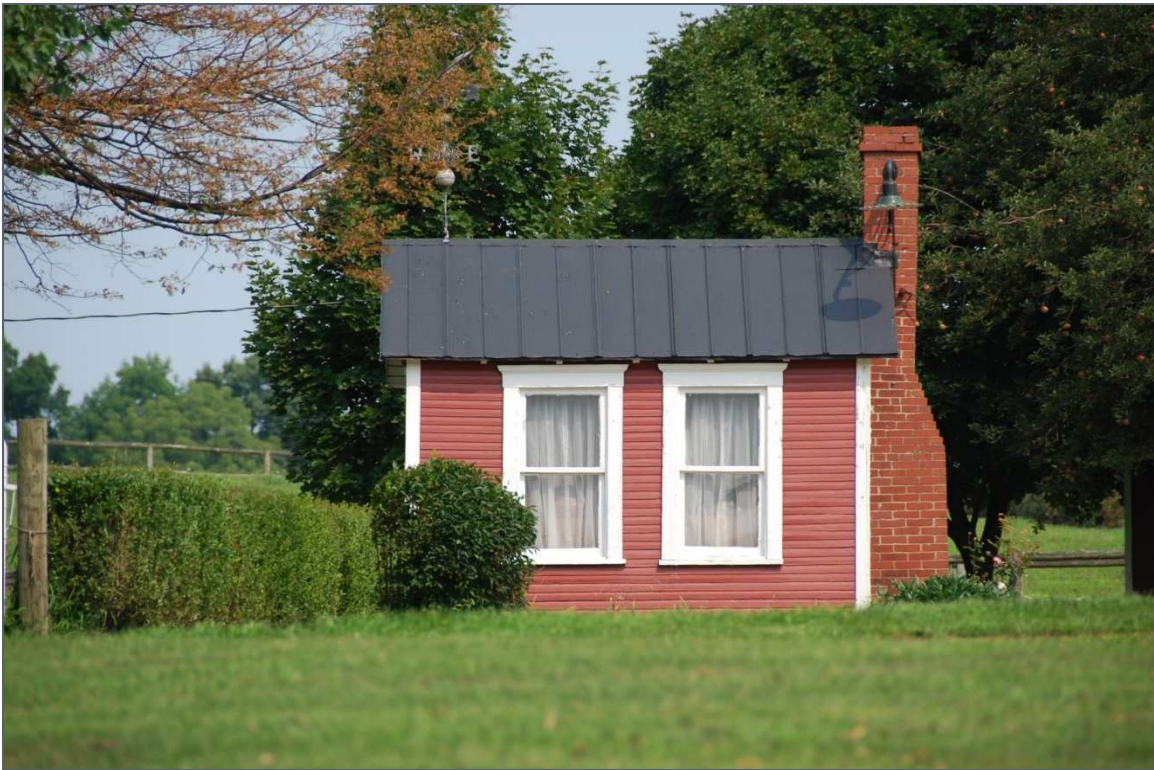
#802074—323 Water Dam Rd., Hickory, Mount Pleasant Township Washington County.
