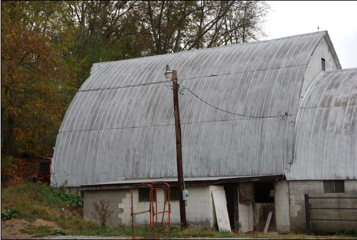
#802501—512 Poplar St., Avella, Buffalo Township, Washington County. A Rainbow Roof barn that appears to have adapted essentially to a Wisconsin Dairy barn as a result of the milking parlor addition.
