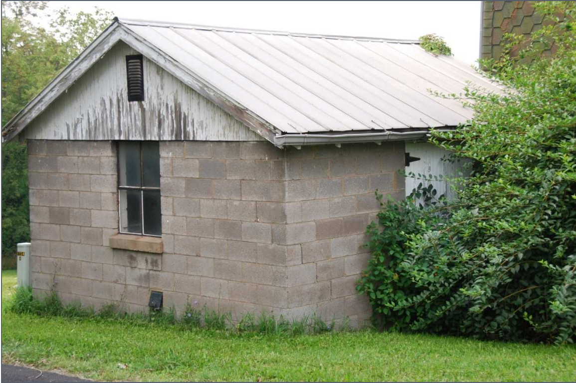
#802083—14 Johnston Rd., McDonald, Mount Pleasant Township Washington County. A concrete block milk house with gable roof.
