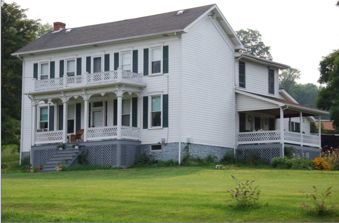
#802099—Muse Bishop Rd., Canonsburg, Cecil Township, Washington County. Example of I-House, 5 bay with later folk Victorian additions, front porch with balustrade, bracketing, spindle work.
