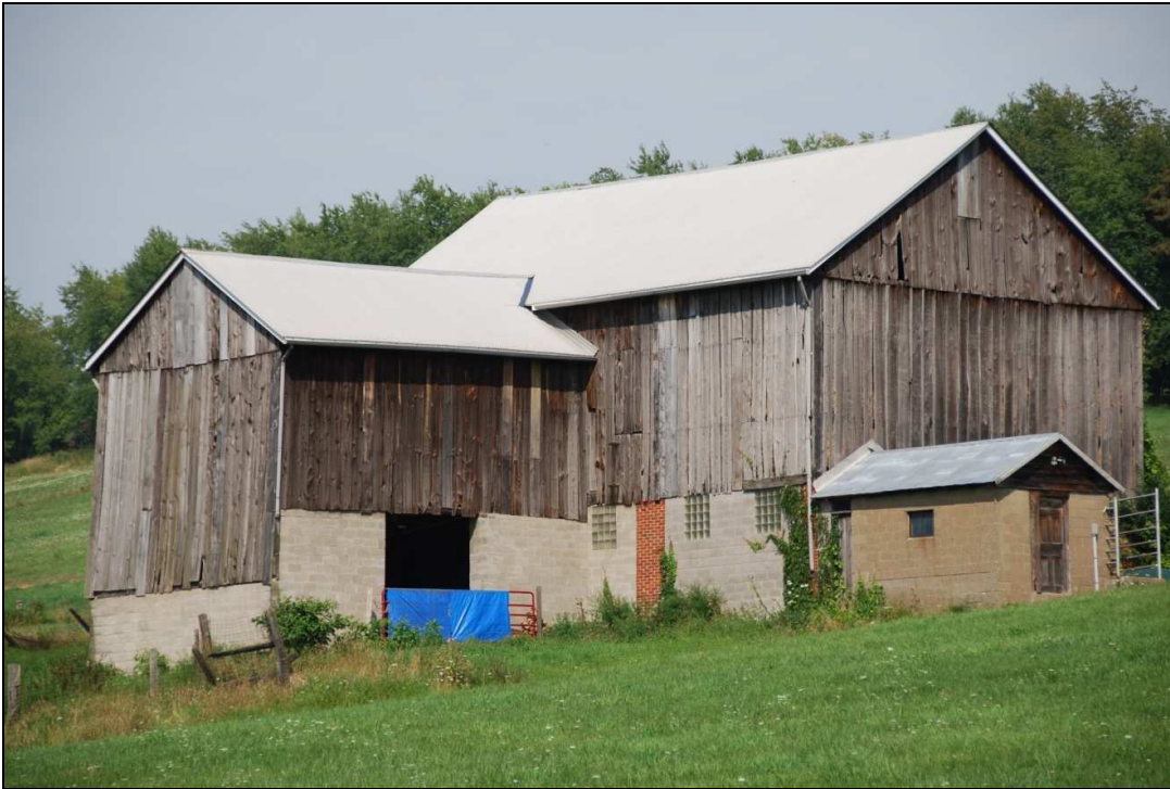
#802062—O.P. Cooke, 1446 N Rt. 18 Hickory, Smith Township Washington County. Notice entry is only to the basement story, there is no access to the upper story by ramp, banking, or a bridge.
