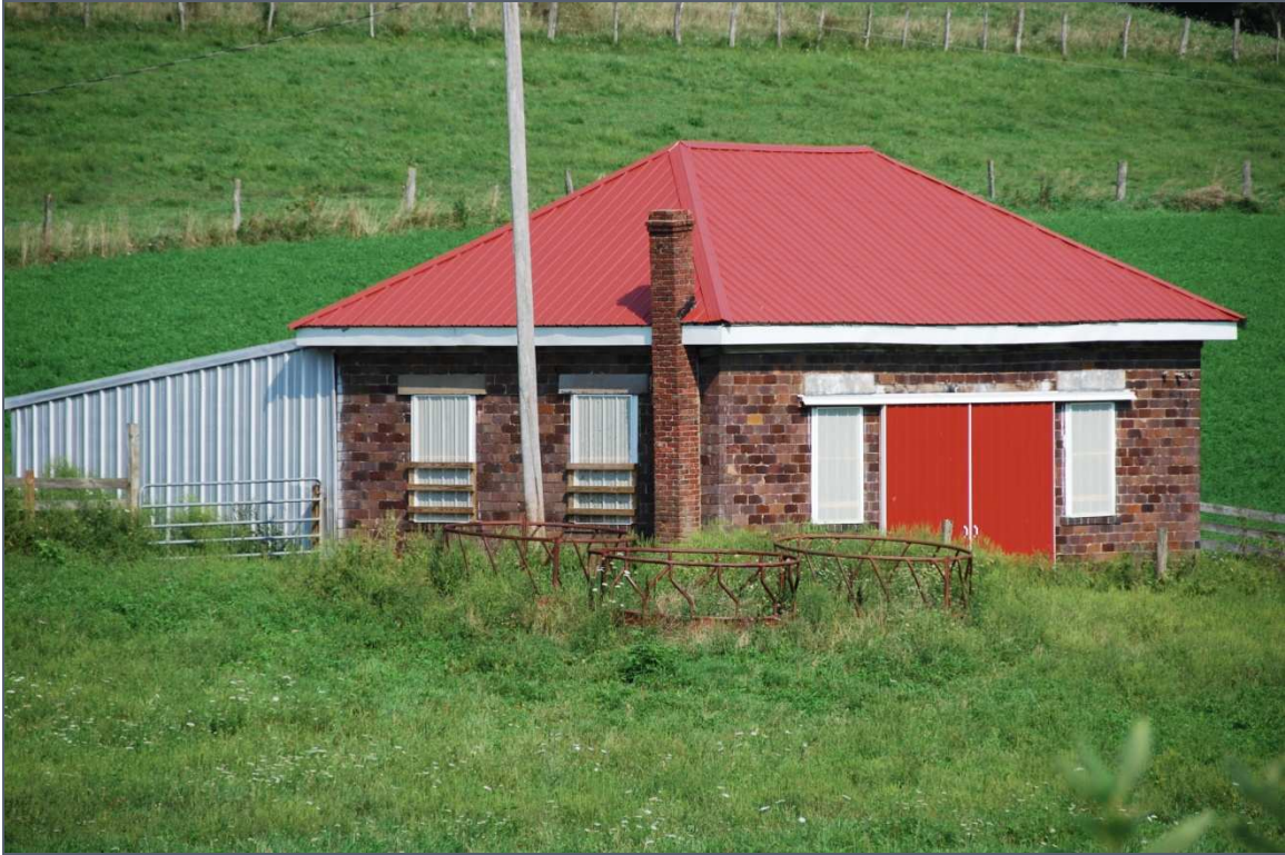
#802130—214 Cedar Grove Rd., Avella, Jefferson Township Washington County. An early 20 th century workshop.
