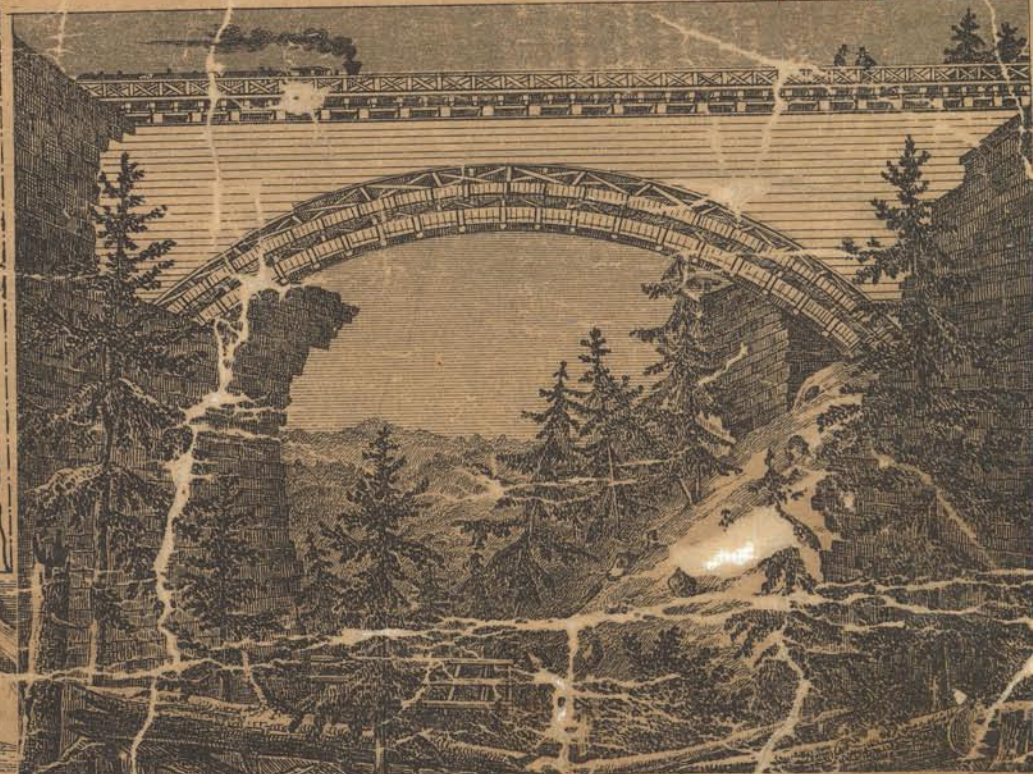
CASCADE BRIDGE On the N.Y. and Erie R.R. near Lansboro.
